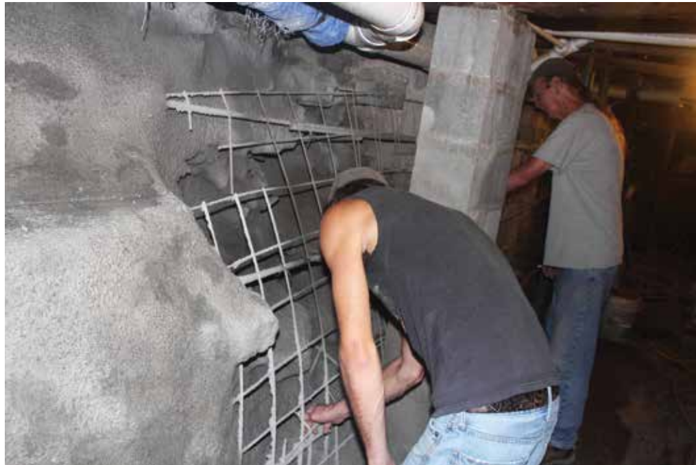
AT WORK: Larry Garlock and Mike Fetter are working on a project at the Village News .
