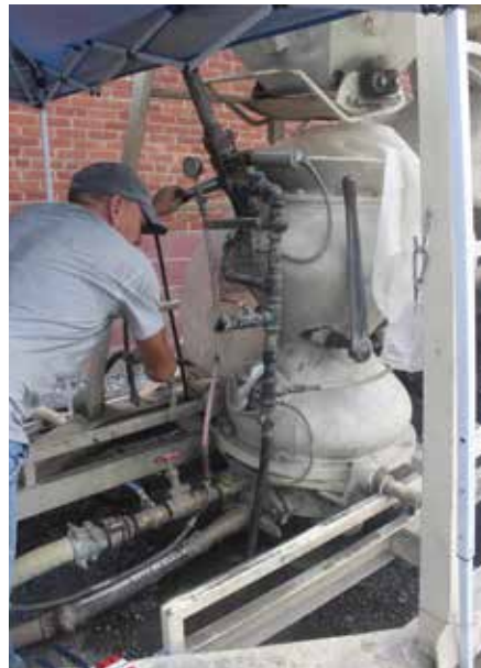
MILLER AT WORK: Bill Miller works with the gunitite-mixing machine he rescued from a junk yard and rebuilt himself.
